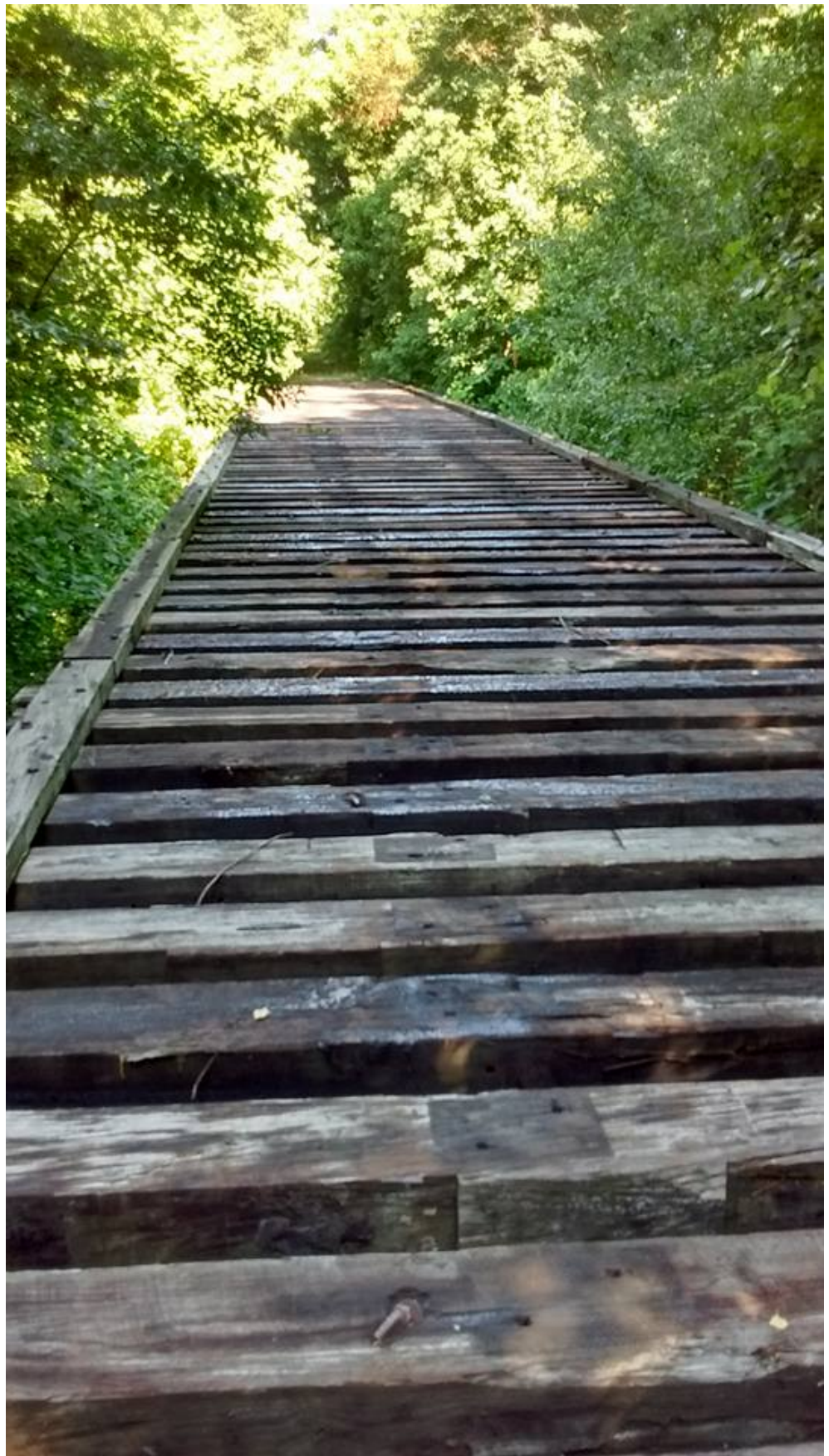
East Bear Creek Trestle Bridge. Photo by Jennifer Holcombe.
